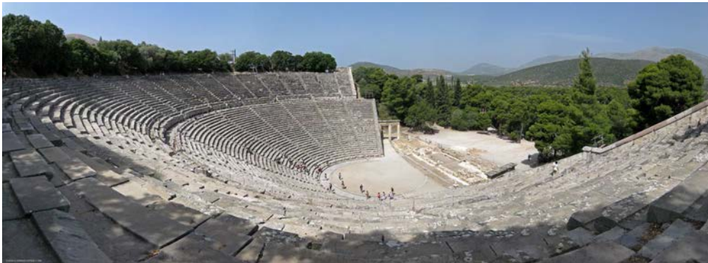
Fig. 3. The Large Epidaurus Theatre: a) ground plan; b) a photograph of the venue (author: Gonzalo Serrano (CC BY-NC 2.0), source: https://www.flickr.com/photos/gserrano22/6961616996/in/photolist-PL5JVq-5yMeg4-bBb7cf-7MPHmt-v7Rov-7MPGQV-6XgnC1-5PirNN-2g9r1Lk-acoooJ-6XgnNC-7MPJG8-duasxJ-duDajZ-7zZRp9-7zW5VT-duDdta-du-JMmS-xZC9Nu-7zZR5o-acoikC ).
